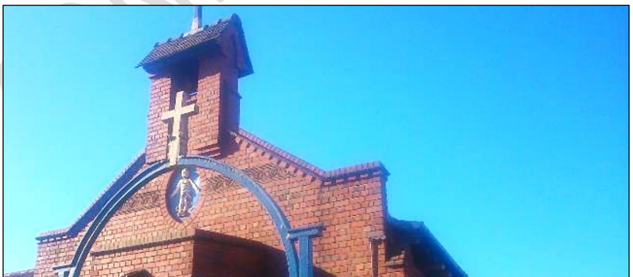
Architectural detailing, St Joseph's and St Theresa's Primary School and Nursery, Chasetown
