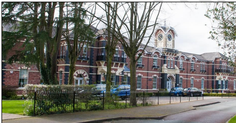
St Matthews Hospital site
